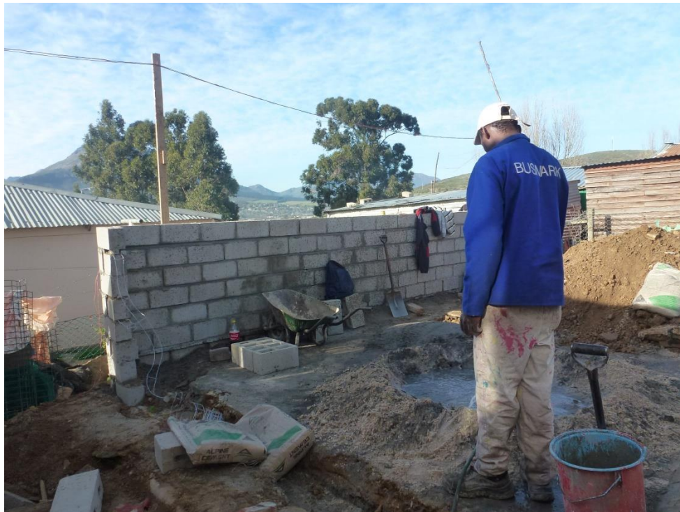
The new crèche taking shape. The loan/grant was used to purchase and install small toilets in the permanent structure
